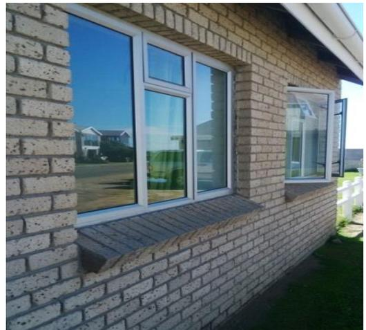
Old wood window frames replaced with aluminium frames at Stywelyne
