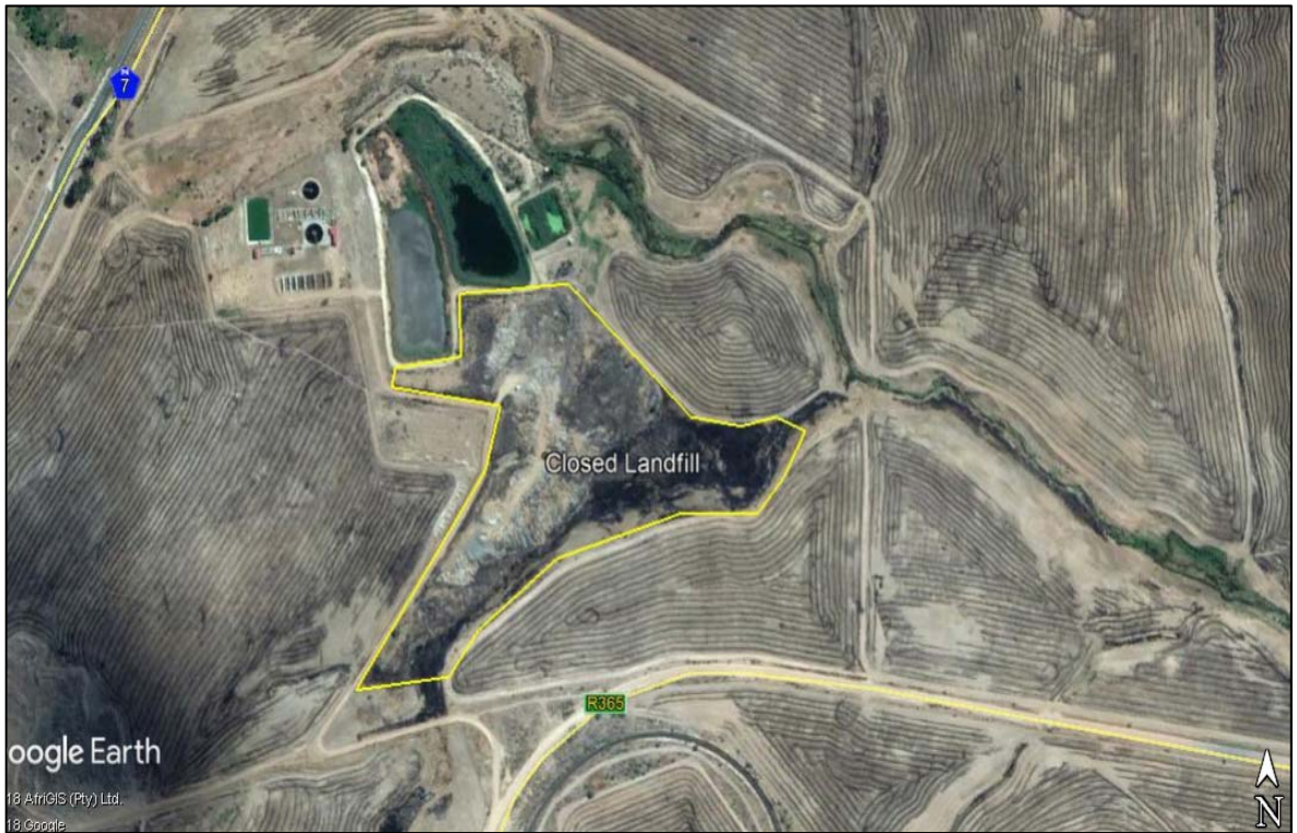
Figure 3.13: Closed Piketberg Landfill
