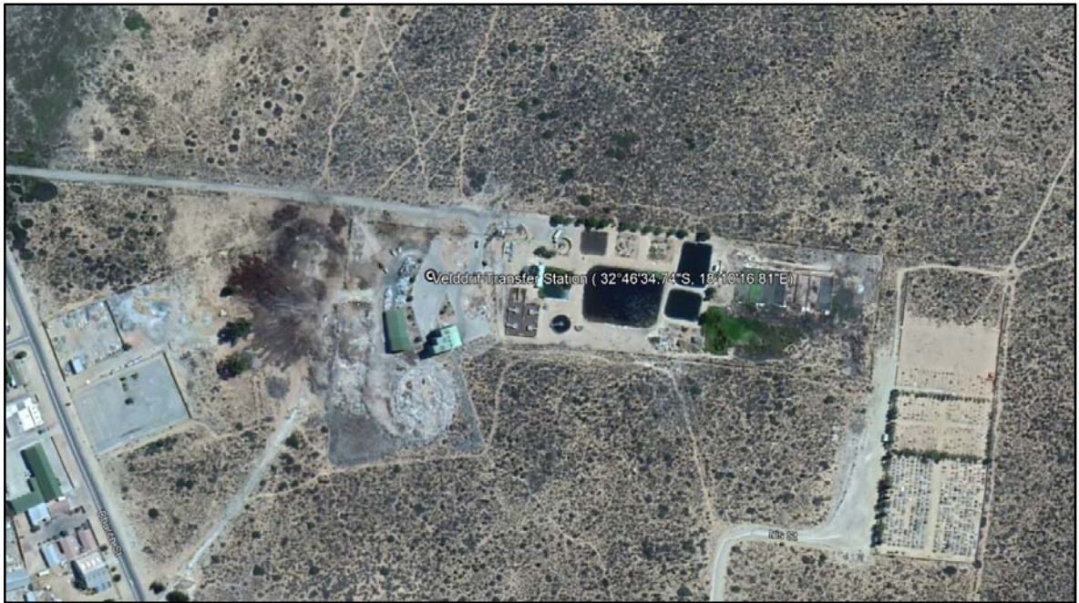
Figure 3.18: Velddrif Solid Waste Transfer Station
